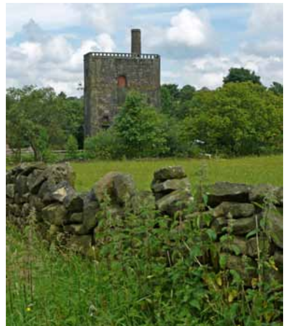
Lumbutts Mill water tower
